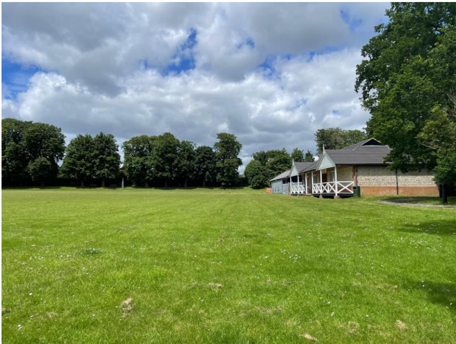
Photo 9. View across modified grassland on Recreation Field.
