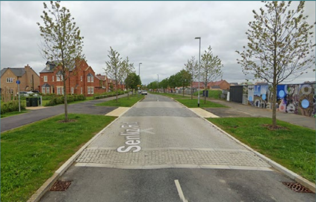
RAISE TABLE TO PRIORITISE PEDESTRIAN & CYCLIST CROSSING - EXAMPLE FOR ILLUSTRATION ONLY
